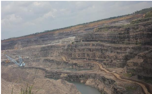
Fig 3: Overview of Sonepur Bazari Project, Eastern Coalfields Limited, CIL, India
