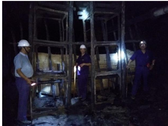
Fig 4: Arrangements for sand stowing with barricades and hydraulic filling of sand in seam #4
