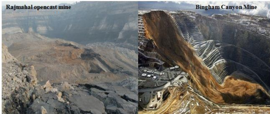
Fig.2 Slope Disaster at Rajmahal opencast mine, ECL, India on 29-12-16 and at Bingham Canyon Mine southwest of Salt Lake City, USA on 10-04-13.
