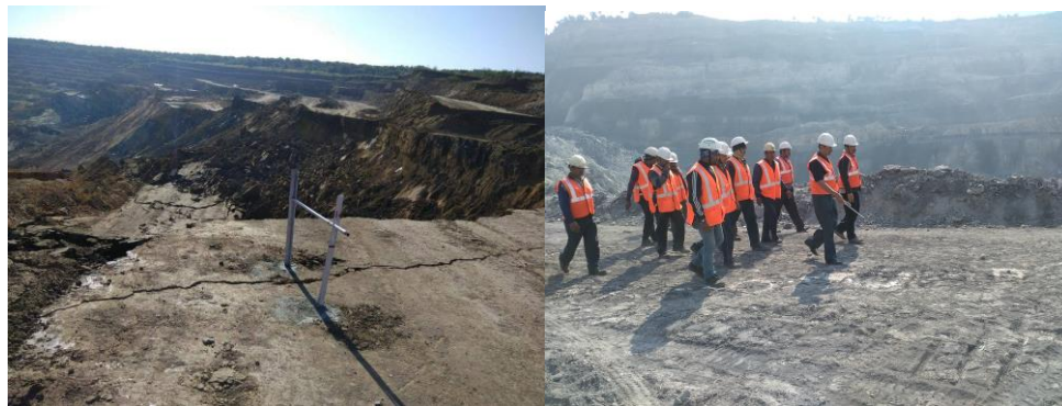
Fig 3: Status of benches in typical opencast mines prone for cracks and failure
