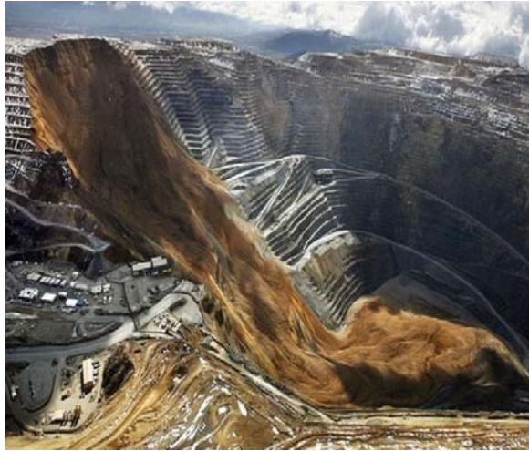
Fig.2b.Slope failure at Bingham Canyon Mine southwest of Salt Lake City [2]
