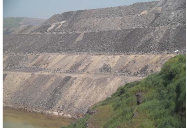
Fig. 6. Decks with Fly ash as admixture in overburden material after compaction
