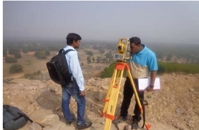
Fig. 11. Total station for measuring Reduced Levels of monitoring stations
