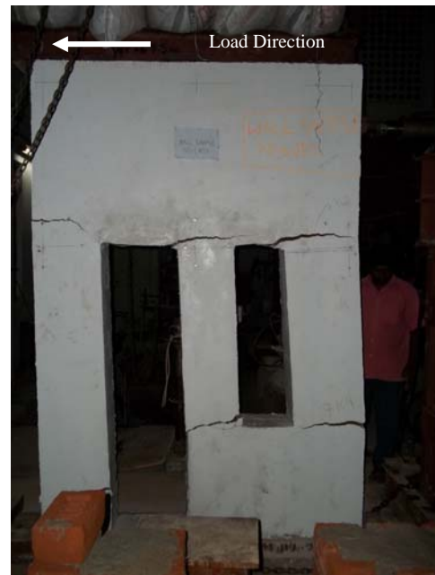
Figure 3. Typical crack pattern of the test specimen (W-10)
