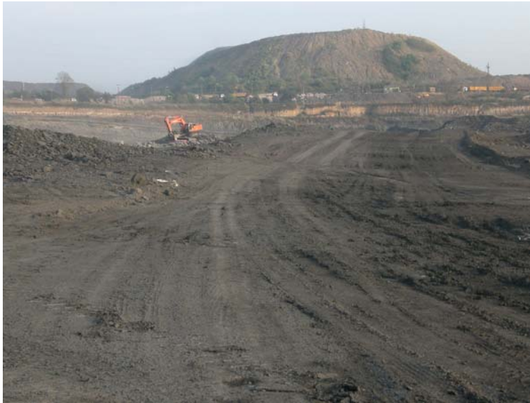
Fig 3: A view of Jindal Opencast mine, Tamnar, JPL
