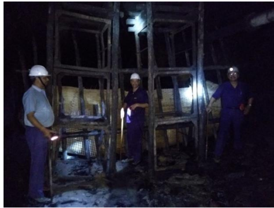
Fig 4: Arrangements for sand stowing with barricades and hydraulic filling of sand in seam #4
