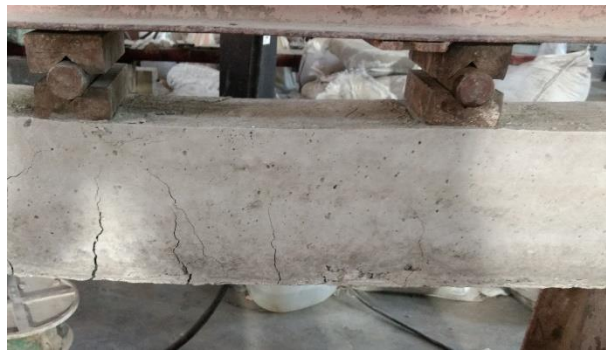
Figure 7: Flexure cracks propagating in RC beam under four point bending test.
