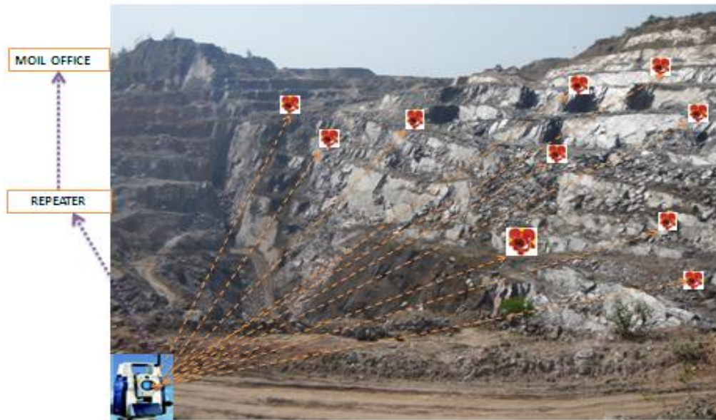
Fig.6. Automatic Total Station Monitoring
