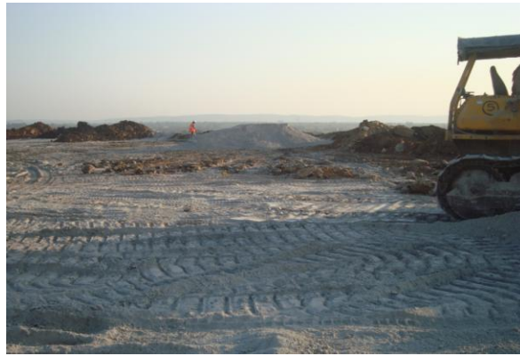
Fig 3: Dozing of fly ash and OB material at the dump site
